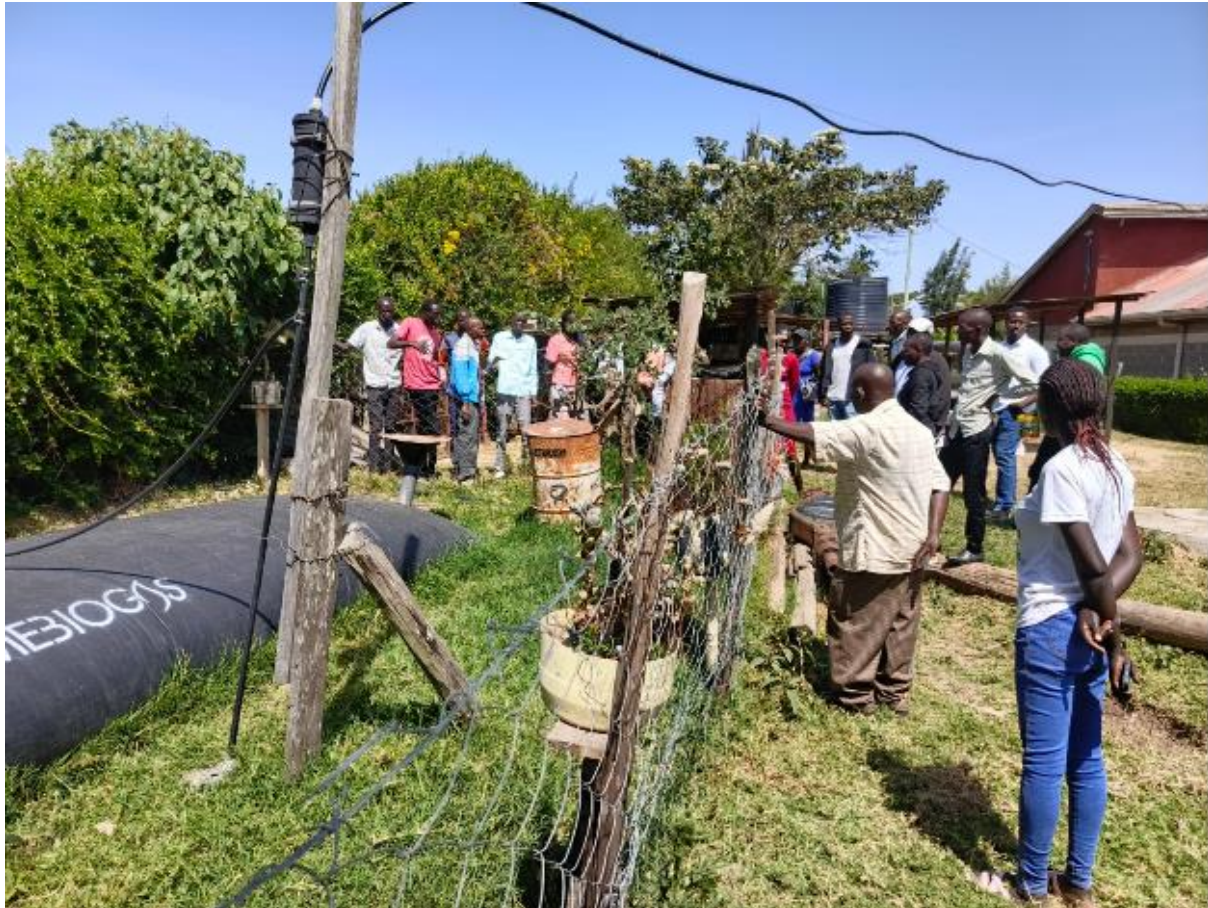
Biogas System at Agnes Farm in Laikipia County
