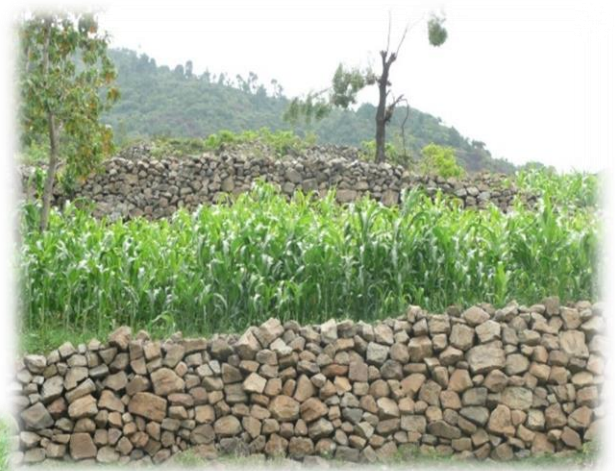
Stone bunding solutions
