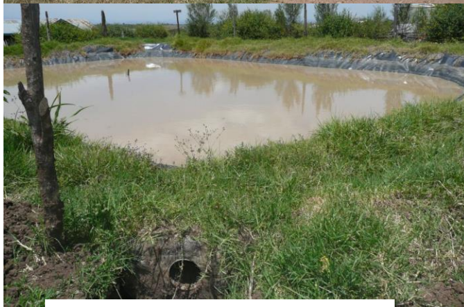
Runoff harvesting with plastic-lined pan
